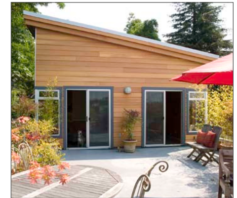
image courtesy PLACE Architects pllc
